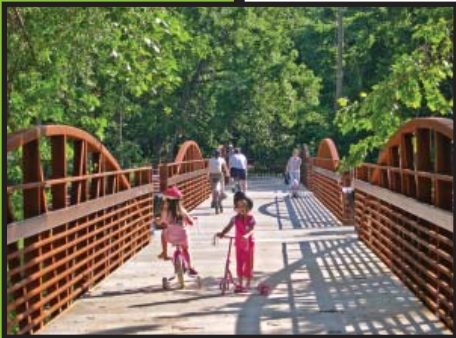
Spillway Bridge Lake Fayetteville
